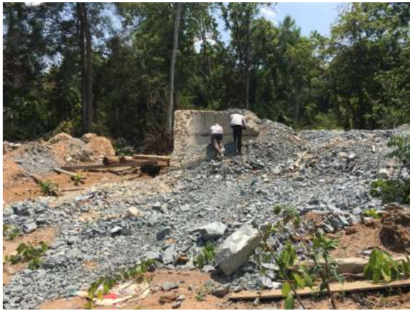
Gold Mining #5. Shaft with concrete casing toward back right of photo. Location marked with rectangle in Section 4a, Figure 5.
